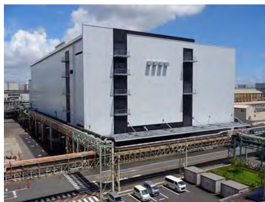
Exterior view of the new plant
